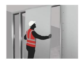
All horizontal joints should be staggered by 300mm, and all vertical joints should be staggered by 600mm as far as practical.
