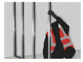
Fix Hadley Resilient Bars across the whole length of the system at maximum 600mm vertical centres and at all perimeters of the wall. Fixing to each stud with wafer head screws.
