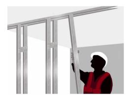
There is no requirement to screw the Hadley C Studs into the Hadley track at the metal framework will become more secure once plasterboard has been screwed in.
